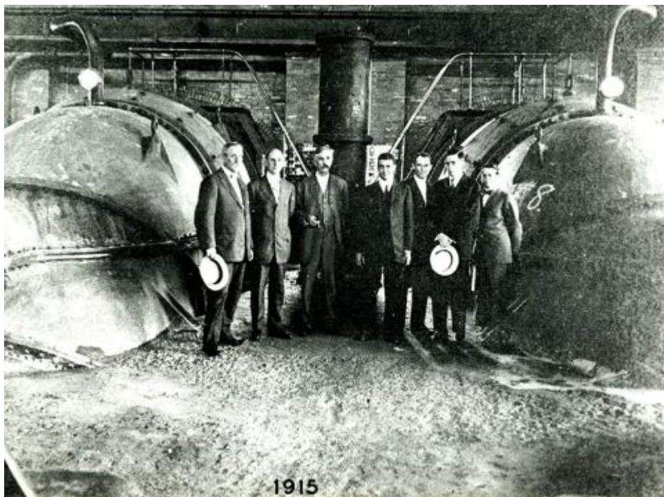
A. Baldwin Wood, center, an 1899 Tulane engineering graduate, is pictured at the 1915 dedication of Station No. 1, which used his revolutionary new screw pump system. Wood invented the pump in the early 1900s, when he was fresh out of Tulane and employed by the New Orleans Sewerage and Water Board. The pumps, more efficient than the centrifugal pumps they replaced, remain in use today, moving rainwater from the streets of New Orleans to Lake Pontchartrain.
